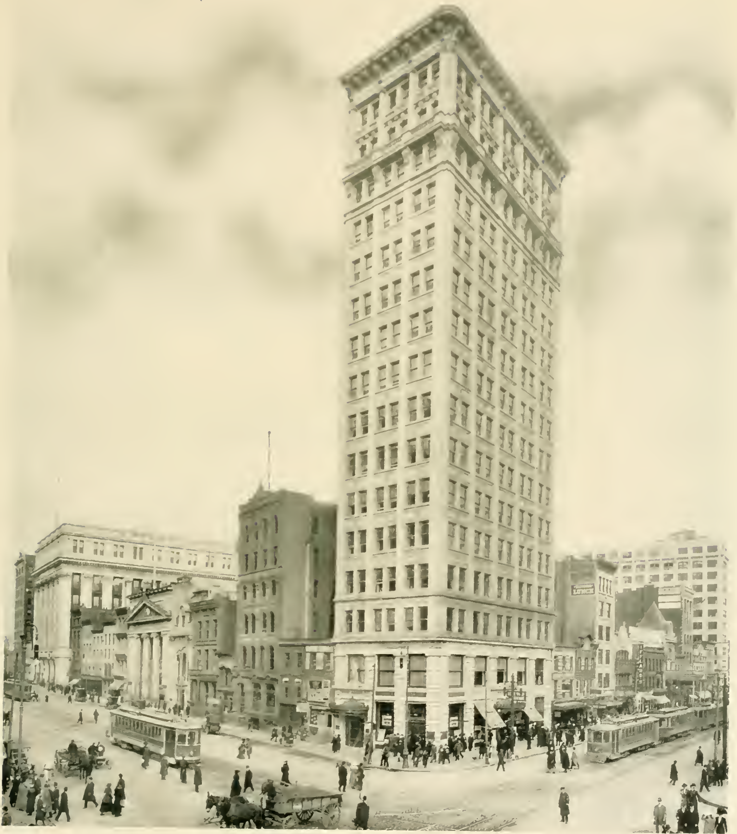
THIS PICTURE IS REPRODUCED FROM A PHOTOGRAPH OF THE NORTHEAST CORNER AT THE INTERSECTION OF BROAD AND MARKET STREETS, WITH THE FIREMEN'S INSURANCE COMPANY'S BUILDING IN THE FOREGROUND. LOOKING TOWARD THE RIGHT IS SEEN THE THOROUGHFARE OF MARKET STREET WITH THE ORDWAY BUILDING IN THE DISTANCE; AND LOOKING TO THE LEFT MAY BE SEEN THE EASTERN SIDE OF BROAD STREET, A SECTION OF NEWARK'S BANKING DISTRICT AND THE MUTUAL BENEFIT LIFE INSURANCE COMPANY'S BUILDING.
